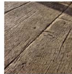
Gilpin's Falls Bridge Plank
