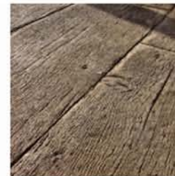
Gilpin's Falls Bridge Plank
